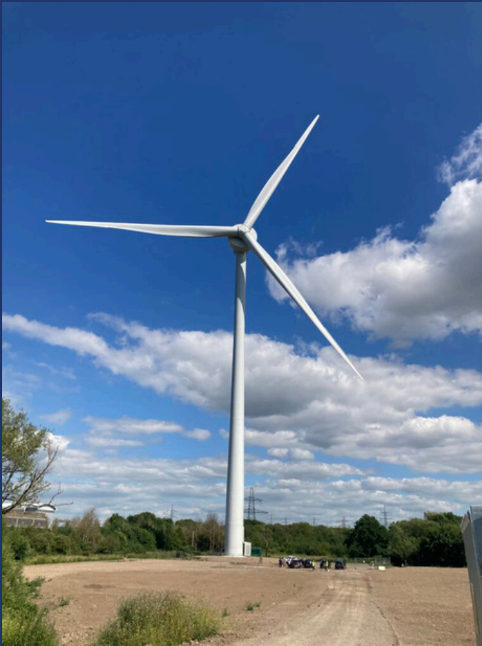
Osprey installed the tallest onshore turbine in England (150 m) to generate clean power for 3,000 homes in Bristol.
